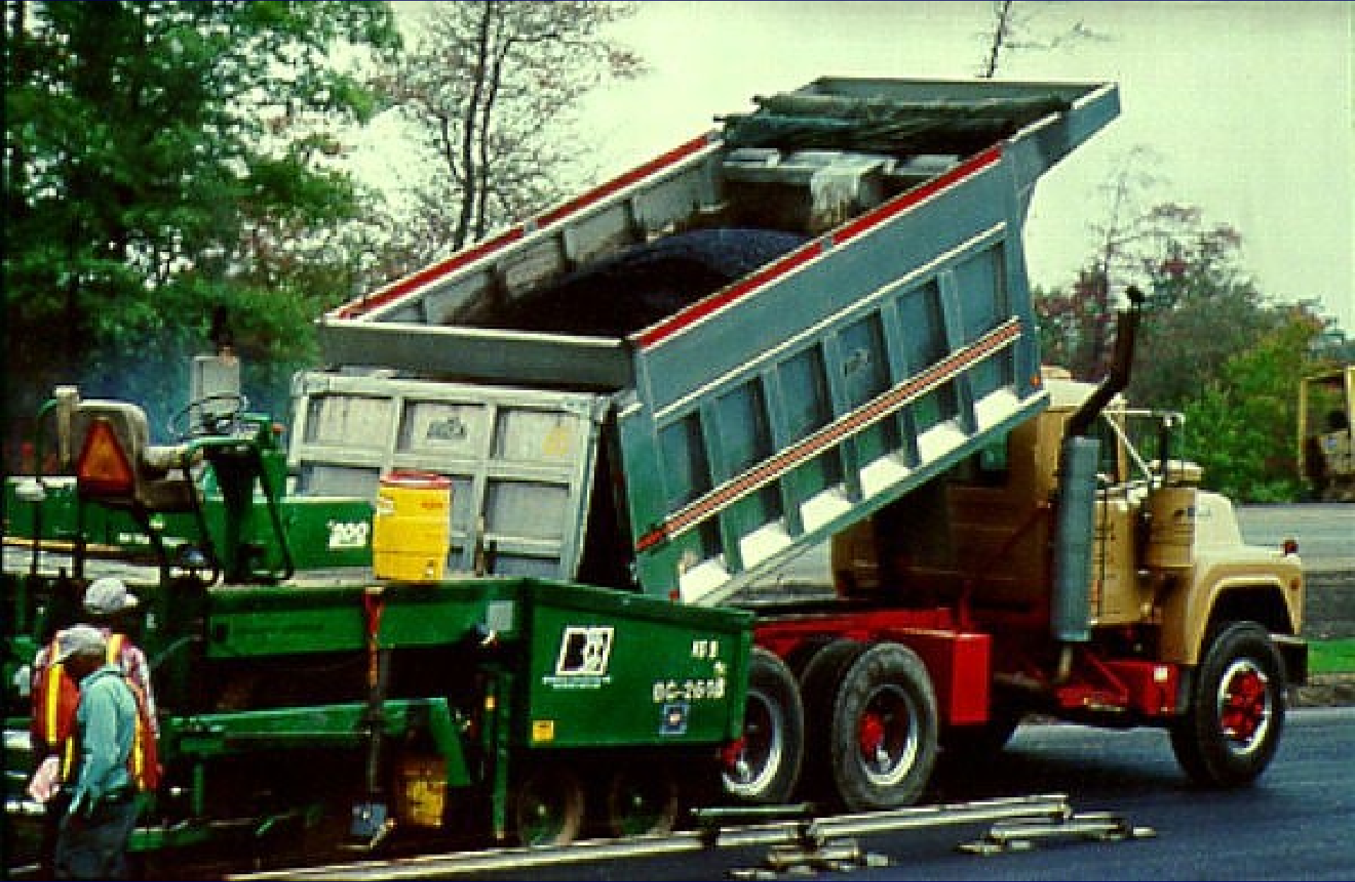
Loading HMA in the Paver
