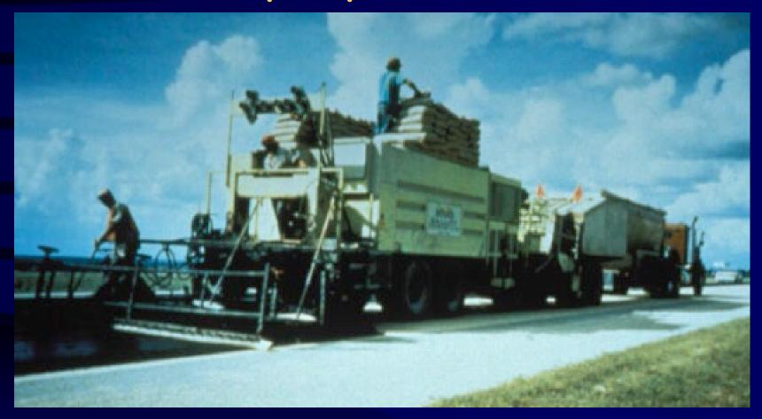
Self-propelled, front-feed, continuous mixing machine
