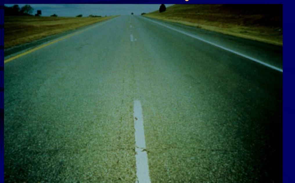
Micro-Surfacing Cost  $\succ$  Unit cost > hot-mix asphalt ➤Cost is offset by Thin layers No appurtenance adjustment Easier traffic control
