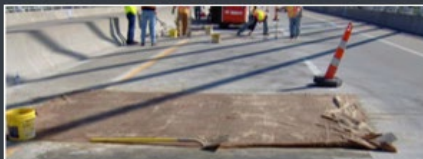
Using Curing Sheets or Mats
