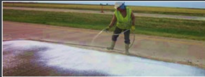
Using Curing Compound
