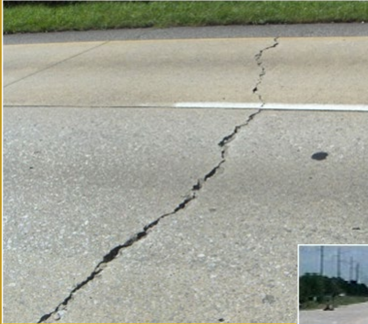
Transverse Cracks
