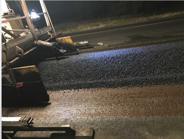
Dense Graded AC (No!)
