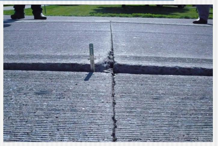
Single lane buckle in a location that was ground when first constructed
