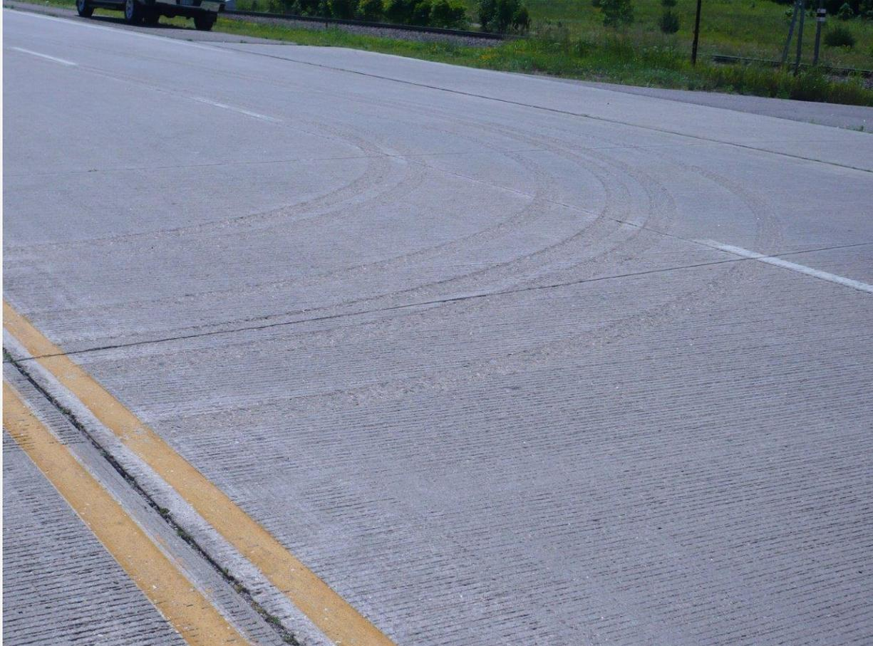
TH 12 Dassel - 25+ year old tracks from vehicle driving on concrete early.
