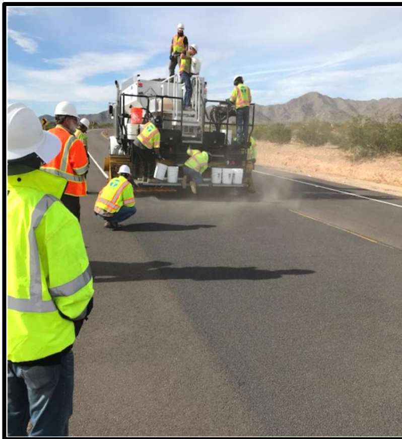
HFST paving operation A fully automated Surface Treatment
