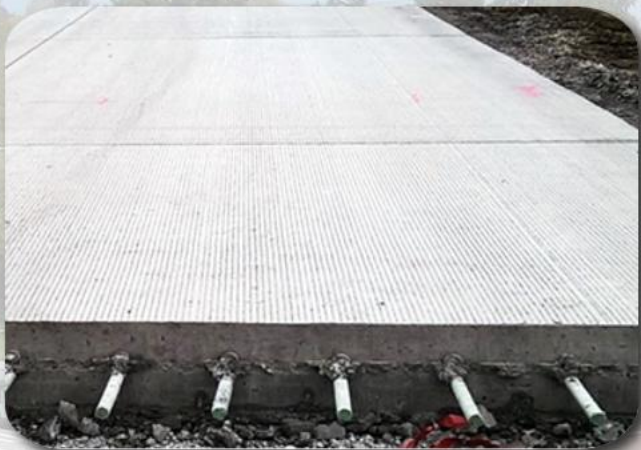
Jointed-Plain Concrete Pavement (JPCP)
