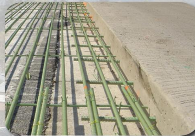
Continuously Reinforced Concrete Pavement (CRCP)
