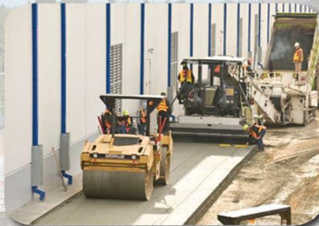
Roller-Compacted Concrete (RCC)
