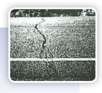
Thermal shrinkage cracking results from either a single thermal cycle where the temperature reaches a critical low temperature or from thermal cycling above the critical low temperature
