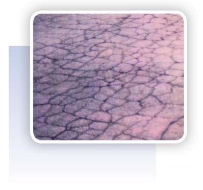
Load-associated fatigue cracking is caused by continuous application of loads over a period of time
