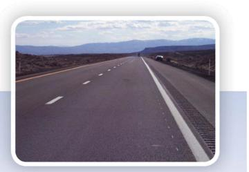
PG 63-22 Modified Asphalt No rutting
