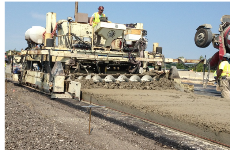
Two-lift concrete construction
