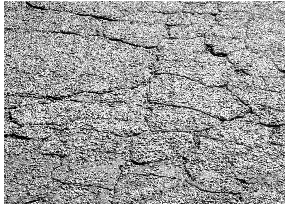
Block Cracking
