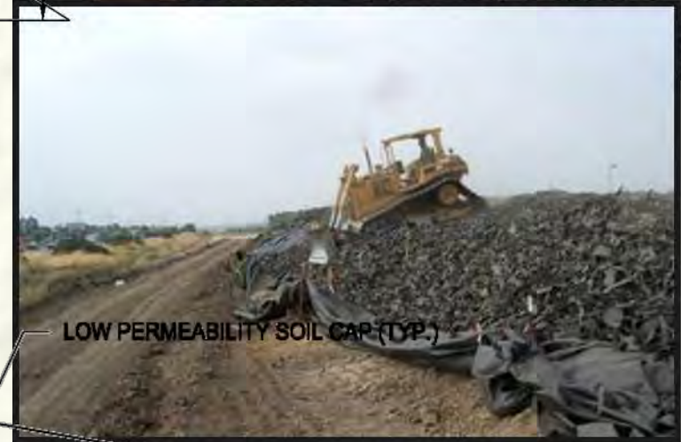
Lightweight Embankment Fill Dixon Landing S880 On Ramp
