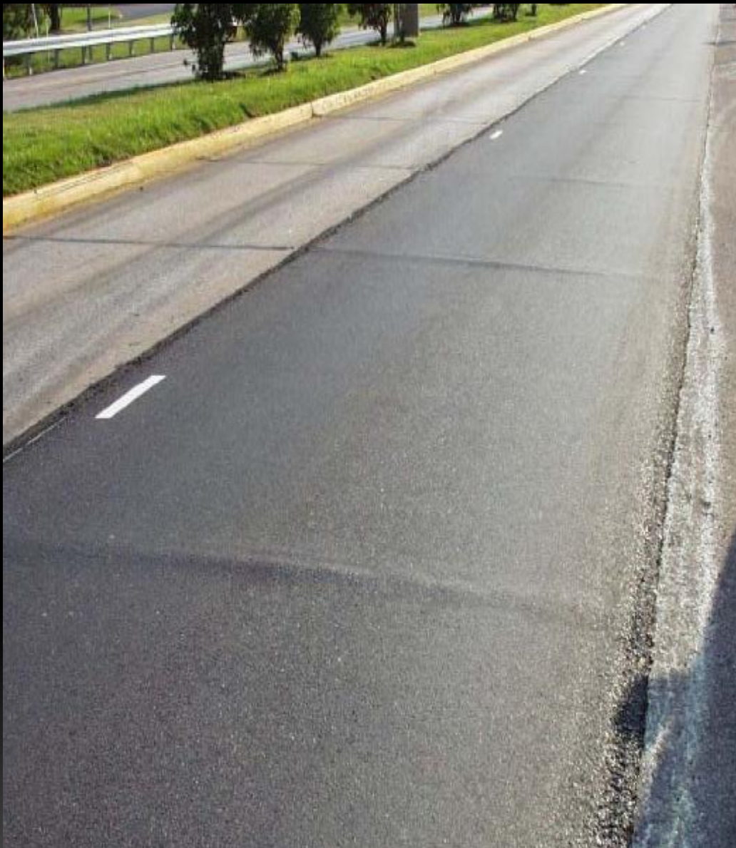
Jointed Concrete Pavement with Rubber Joint Seal Material under HMA
