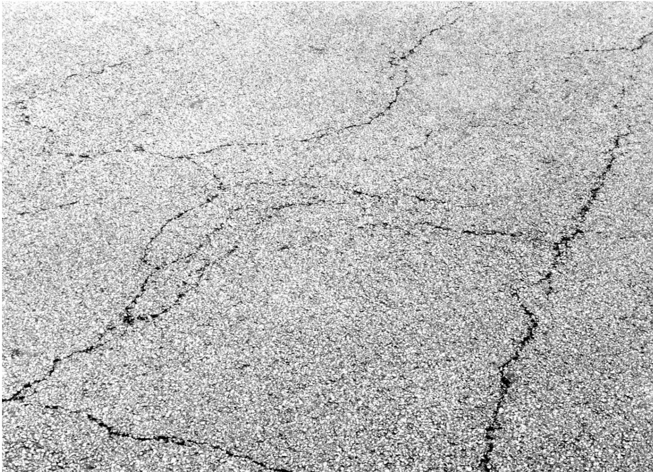
Block Cracking
