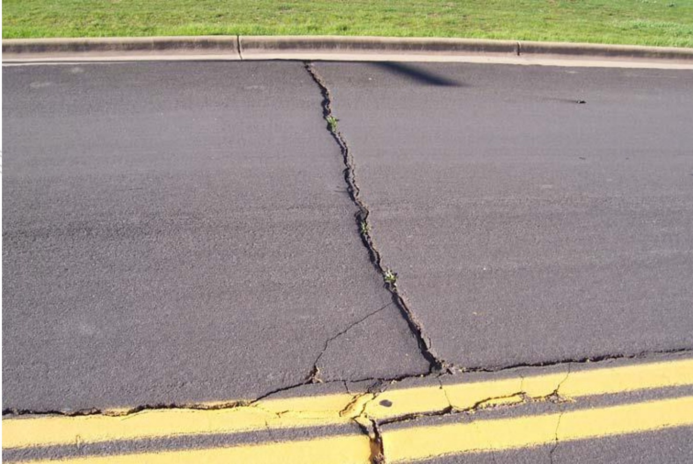
Transverse Cracking
