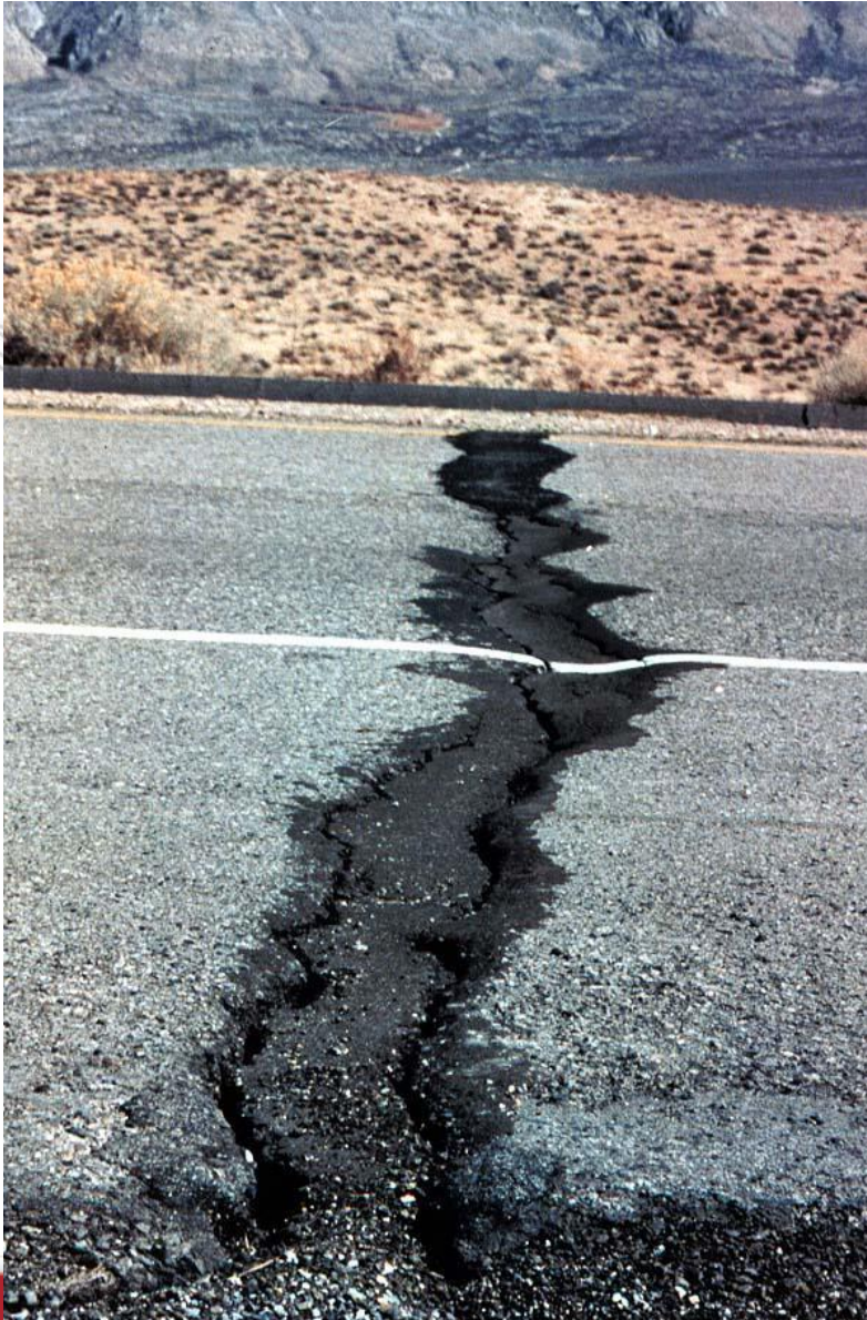
Transverse Cracking
