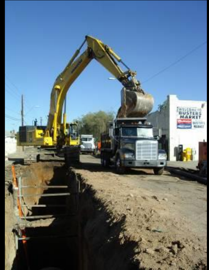
Open Cut Construction
