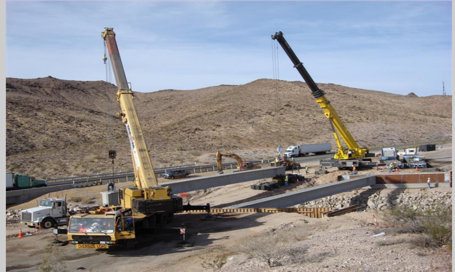
Precast Abutment & Girder Placement
