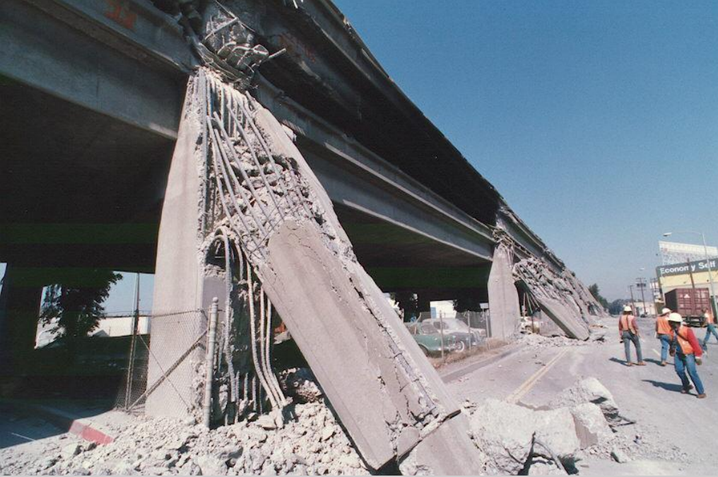
Concrete Viaduct Collapse during the 1989 Loma Prieta Earthquake
