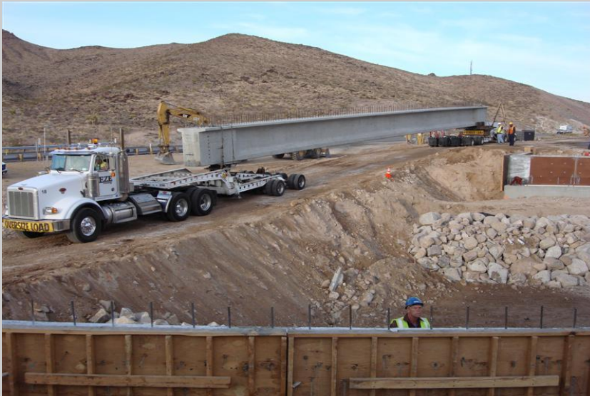
Precast Abutment & Girder Placement
