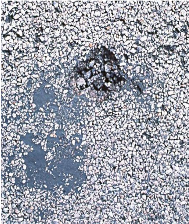
Small pothole with flushed binder on the surface – a sign of moisture damage
