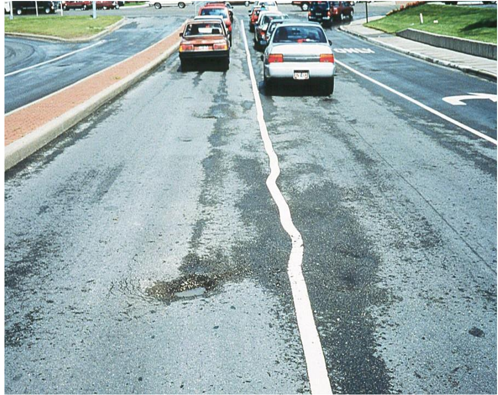
A 1.5" overlay less than one year old that was placed on a layer that was weakened by moisture damage.
