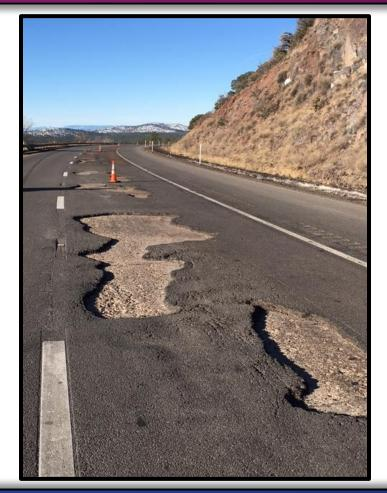
Asphaltic Concrete Overlay on 8 to 9 inch PCCP
